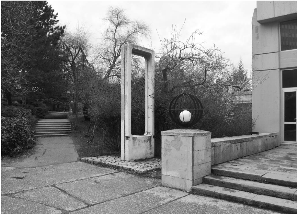
Figure 59. Cafeteria Ground Floor Entrance, Concrete Frame
