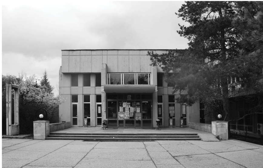
Figure 56. Cafeteria Ground Floor Entrance, photograph by the author, 2022
