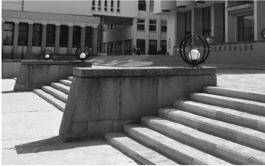
Figure 105. Rectorate retainign wall and lighting unit, photograph by the author, 2022
