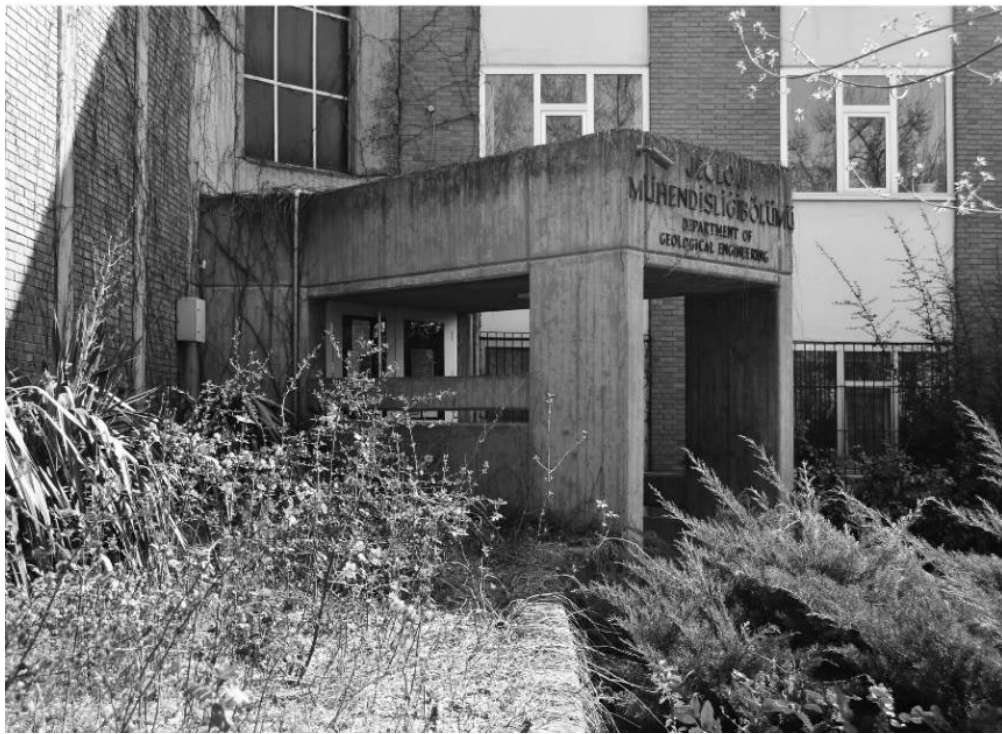
Figure 178. Geology Engineering back entrance, photograph by the author, 2022
