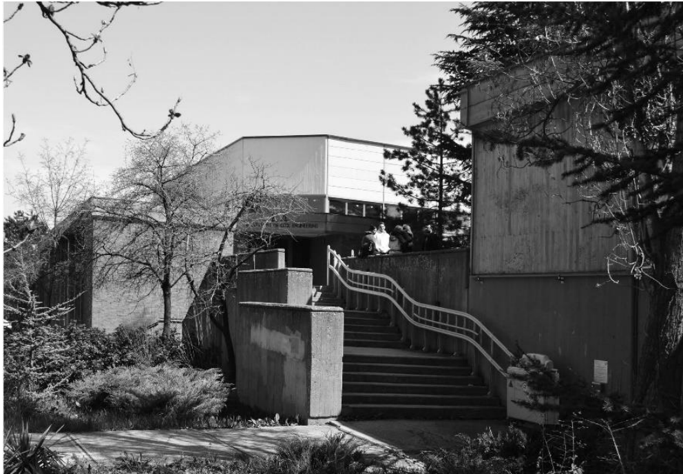
Figure 171. Environment and Civil Engineering buildings complex stairs, photograph by the author, 2022
