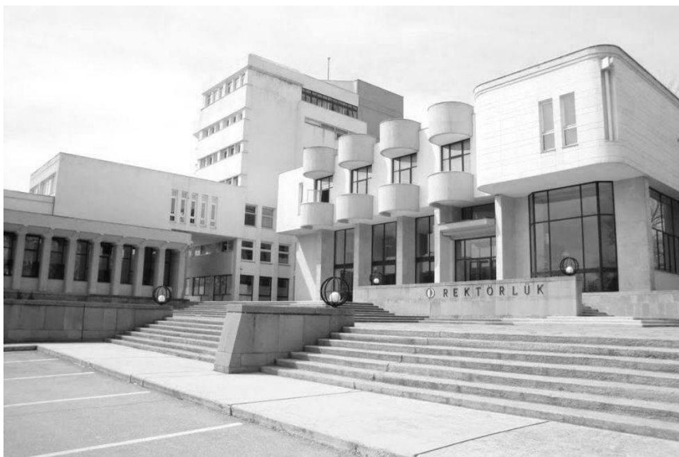
Figure 95. Rectorate building complex, photograph by the author, 2022
