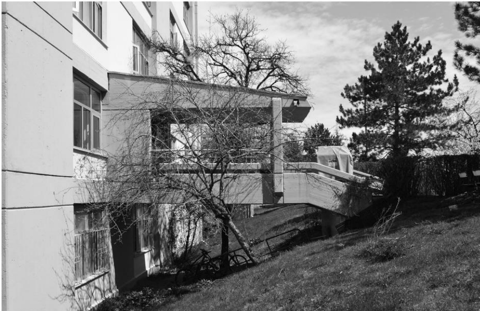
Figure 48. 8th Dormitory Entrance Gate, photograph by Uzay Doğan, 2022
