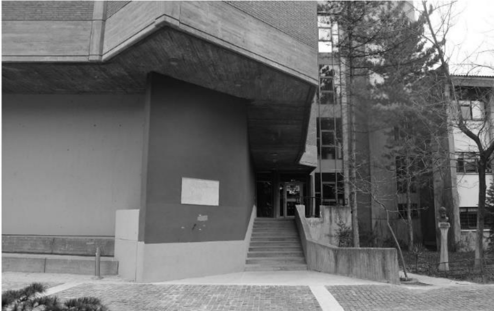
Figure 142. Electric and Electronics department D block entrance, photograph by the author, 2022
